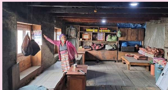
➤ A Sherpa lady switching on the solar light after installation at her house.
