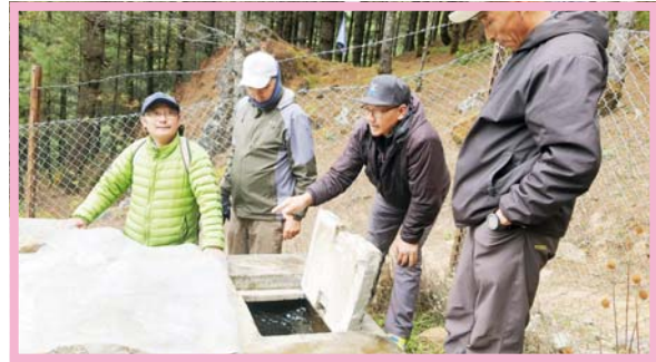
➤ Visit to the Monjo Drinking Water and Fire Hydrant project site.
