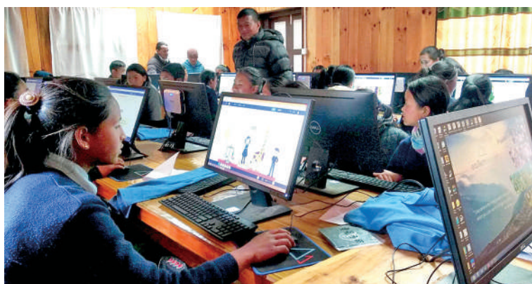
Students using the computer lab after installation of solar power system at Junbesi School
