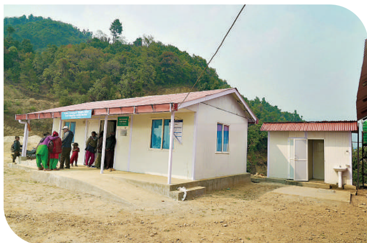
Newly built Patle Community Clinic and toilet.
