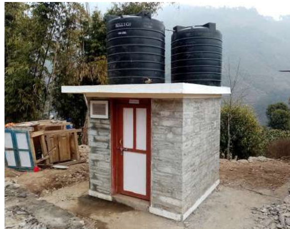
Toilet with water supply in Chomolungmo Basic School
