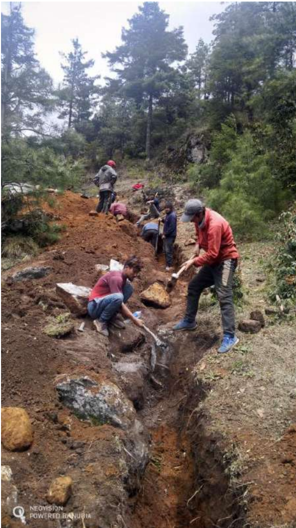
↗ Local youths working for the pipeline trench.
